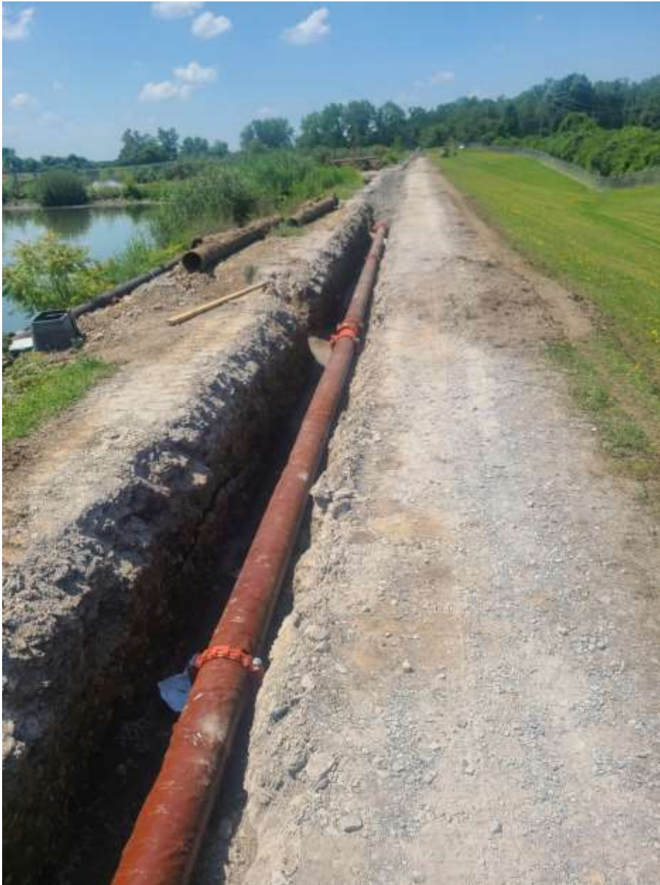
Newly installed pipe with corrosion resistant wrap and high temperature gaskets.
