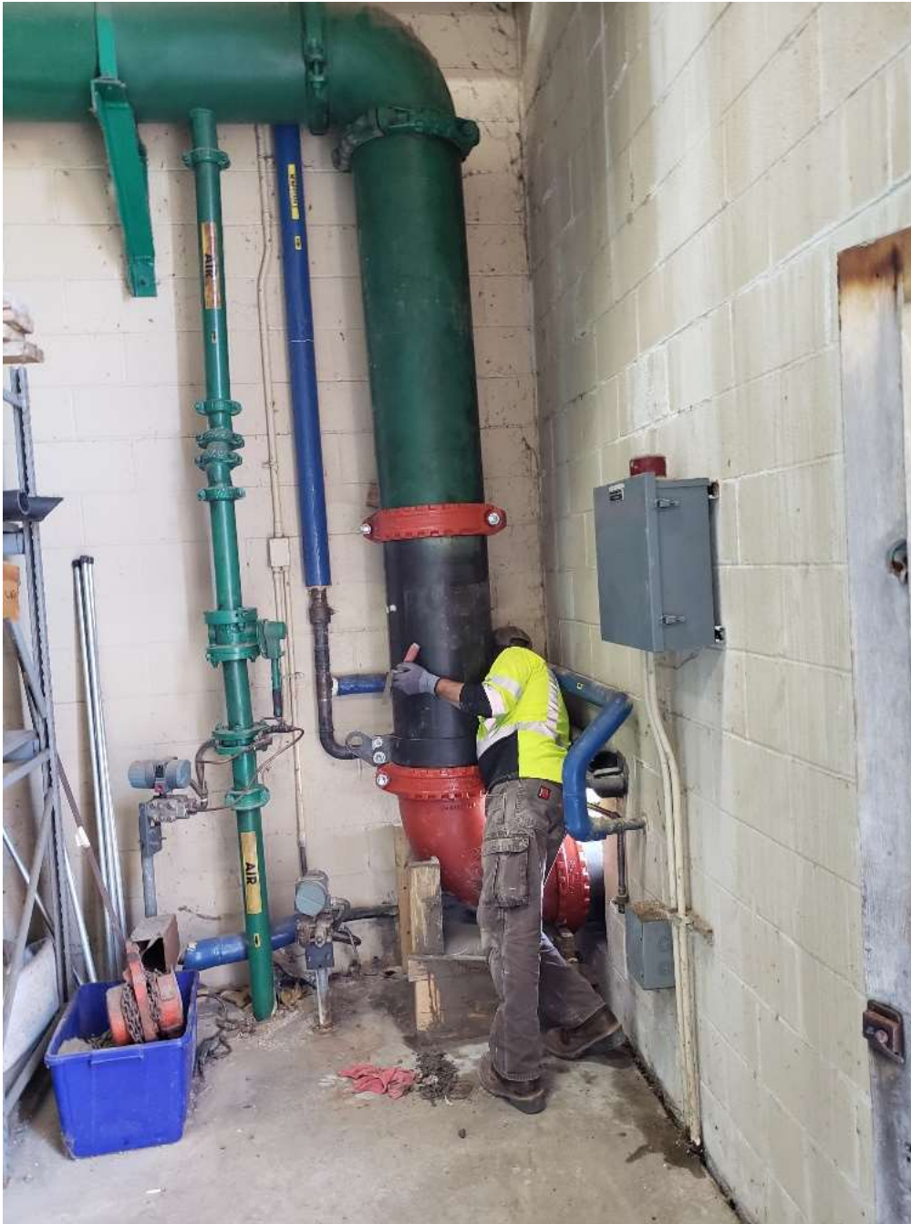
New pipeline being connected to the air compressors.
