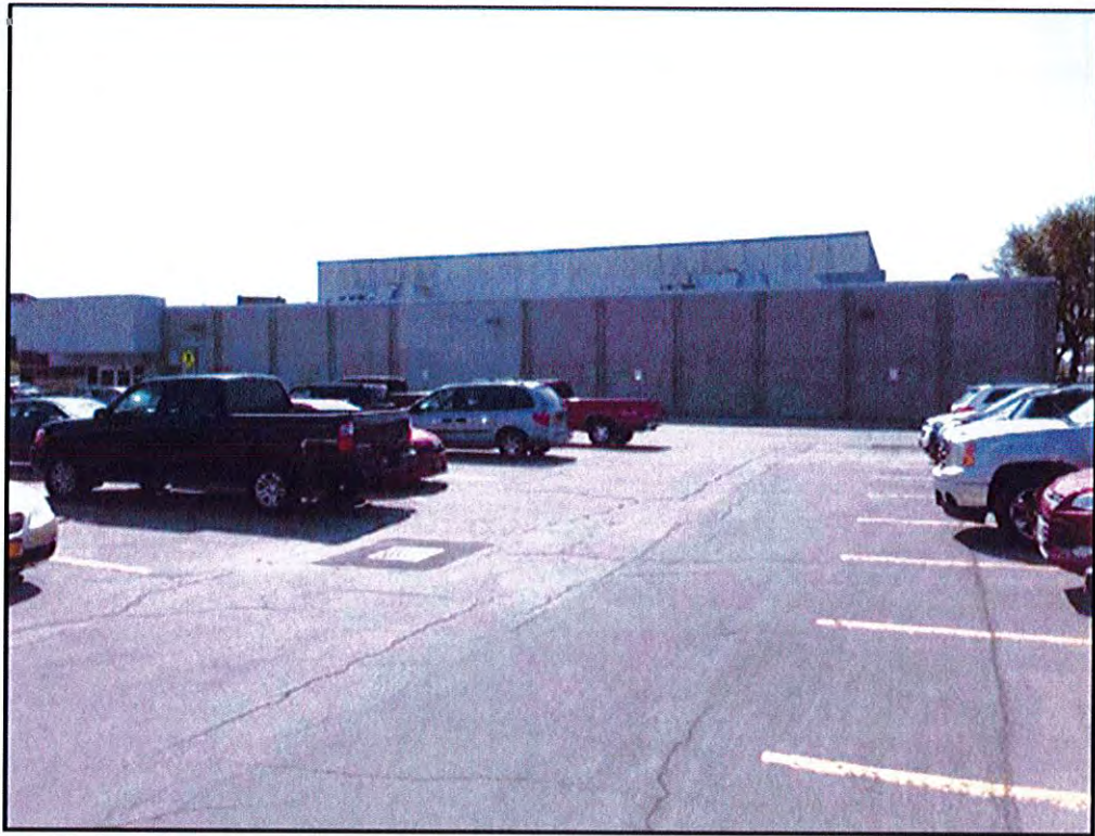
VIEW OF 45-47 ELLICOTT ST. FROM CITY PARKING LOT (COURT ST. SIDE)
