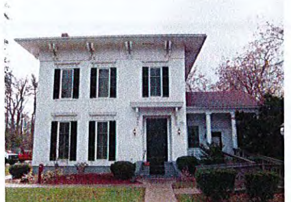
PHOTOGRAPH OF EXISTING NORTH ELEVATION (TO REMAIN AS IS, NO NEW WORK)
