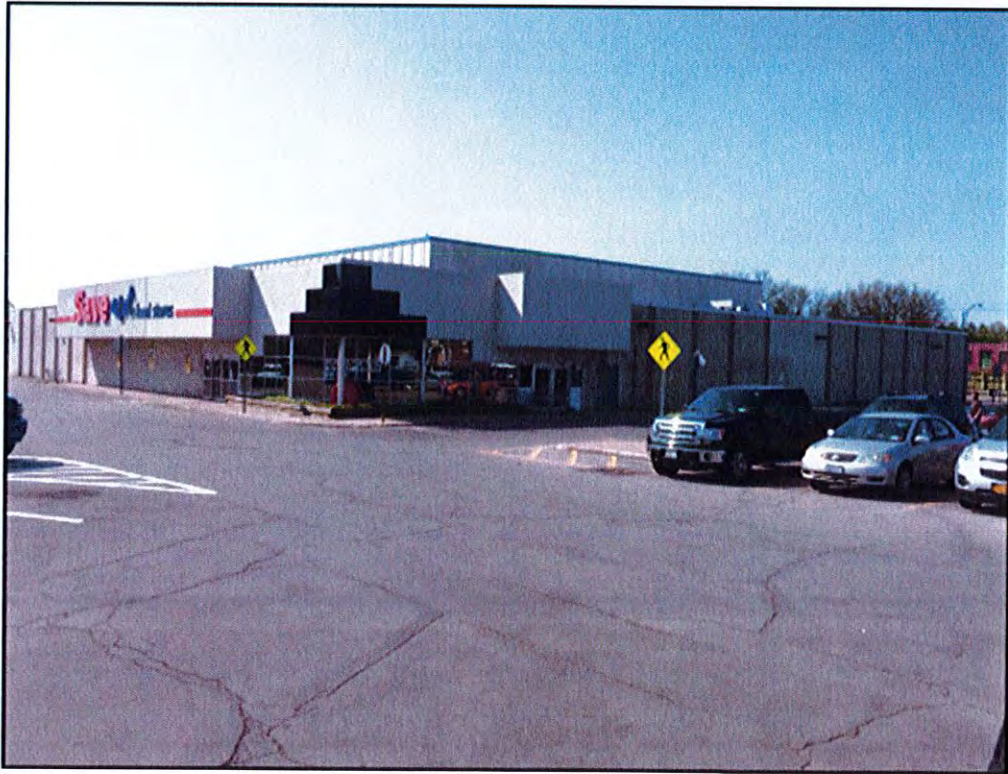
VIEW OF 45-47 ELLICOTT ST. FROM CITY PARKING LOT (M&T BANK)
